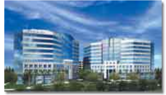
Metroplex Office Centre
