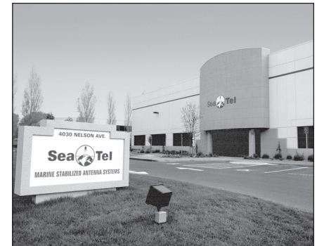
Sea Tel recently expanded into 50,000 square feet in North Concord
